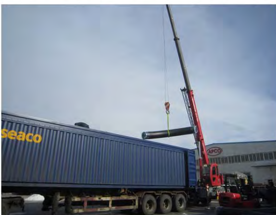
Hot Induction Bends Being loaded
